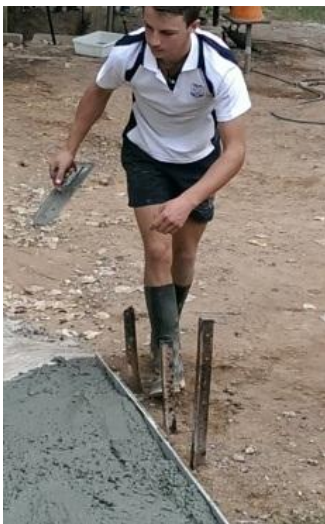
Travis laying concrete
